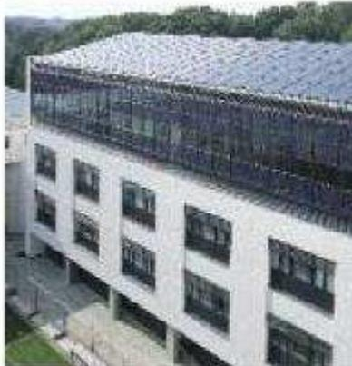
grid-connected BIPV system on the roof and facade of a commercial building.
