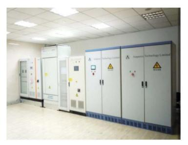
Capacity: 100 kW / 200 kWh Type: PV + Storage + Diesel
