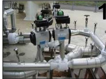
PHOTO 1: ball valves for cryogenic service (oxygen, nitrogen, liquefied natural gas)
